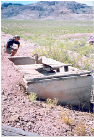
This shaft is 150 ft deep and connects to a large, multi-level stope system.
