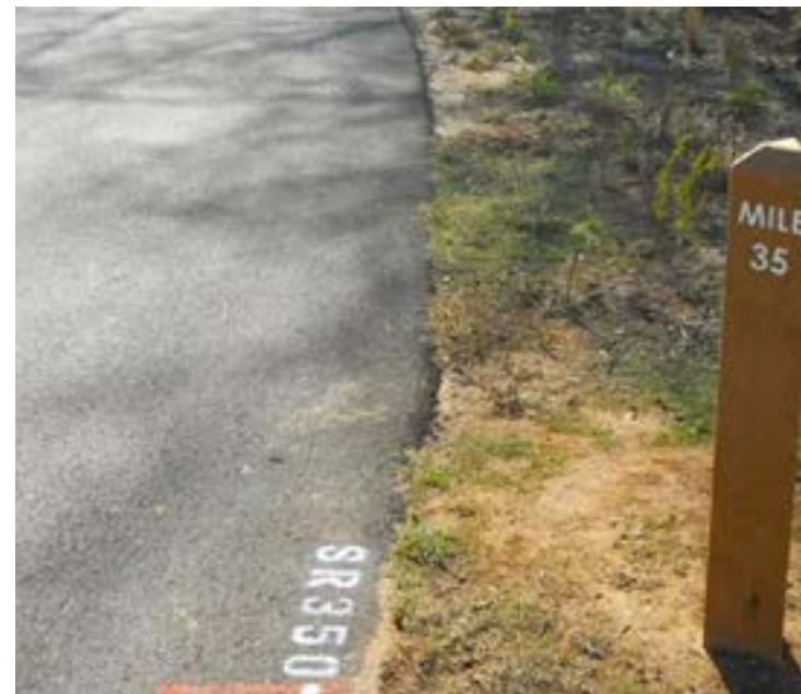
An example of emergency access mile markings (Swamp Rabbit Trail, Greenville, SC). Source: www.FoxCarolina.com
