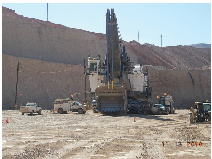
Active mining in 5A Stockpile Area, Tyrone mine, part of the expansion of the West Main Pit, Grant County (2019)
