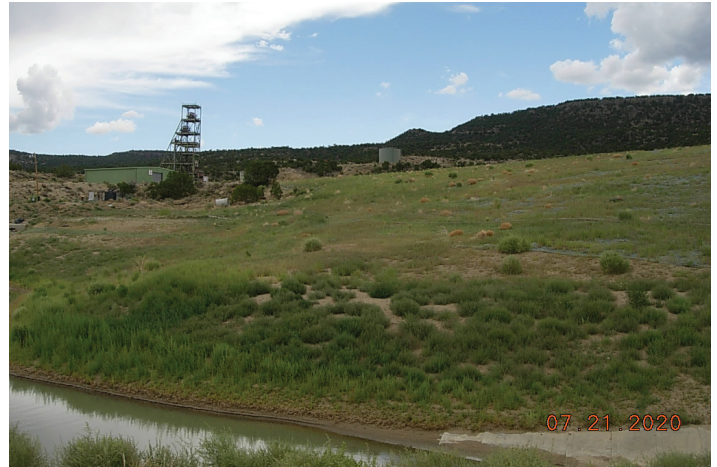
Reclamation has begun at Mt. Taylor Mine. The South Waste Rock Pile has been covered and revegetated, Cibola County (2020)
