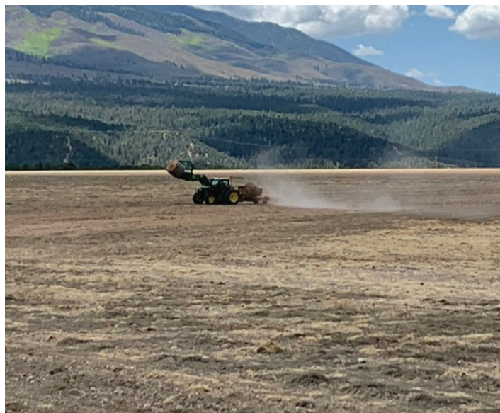
Seeding and mulching at Dam 1 tailings pond reclamation at the Questa Mine, Taos County (2020)
