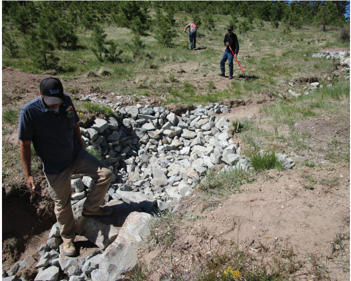
Zuni Bowl construction to remediate headcut, 2019
