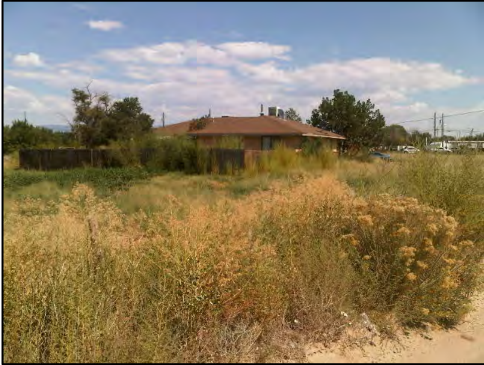
Figure 4-6. Structure requiring defensible space and weed abatement.
