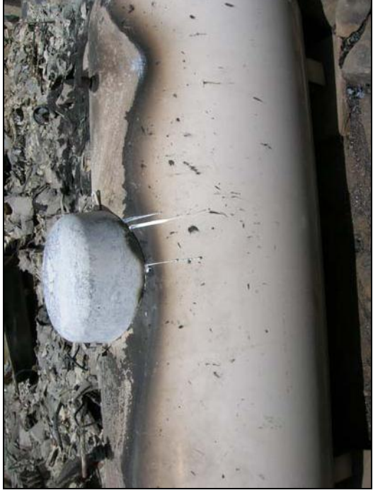
Leaking propane tank. Source: Sam Amato, USFS
