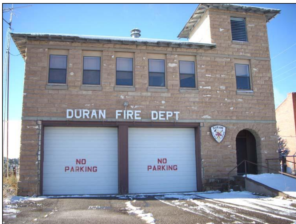
Figure 4.7. Duran fire department.
