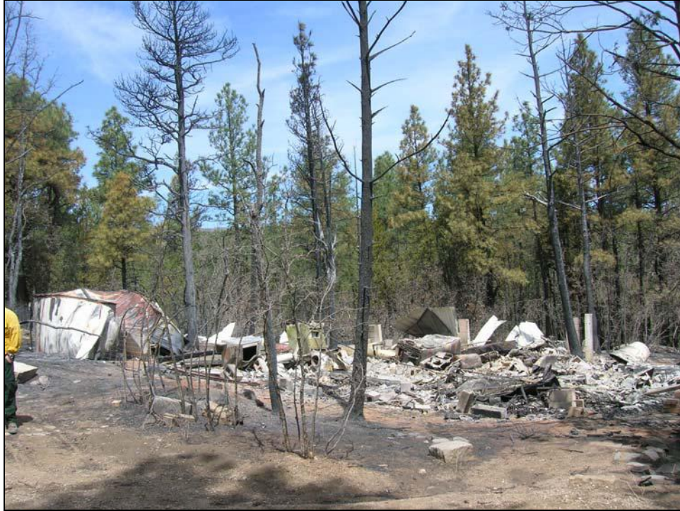
Figure A.14. Green trees with minor scorch surrounding lost structure in Sherwood Forest. Source: Sam Amato, USFS
