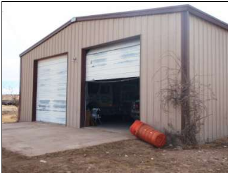
Figure 4.7. Rio Felix fire station.
