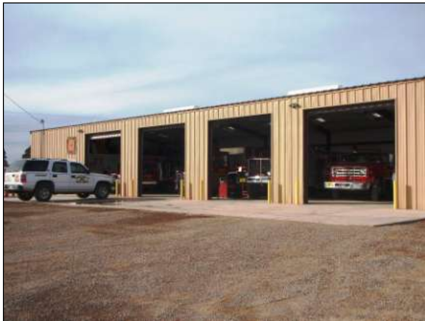
Figure 4.10. District 8 fire department.
