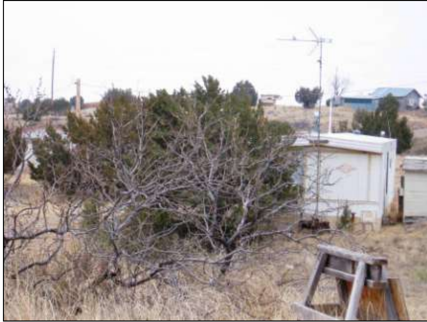
Figure 5.2. Structure requiring defensible space and fuels mitigation.
