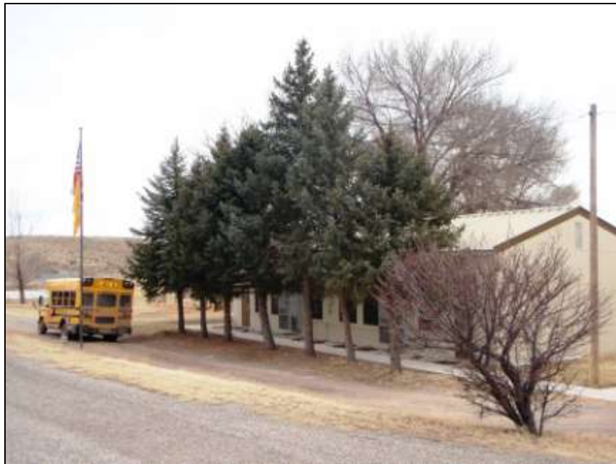
Figure 4.9. Elementary school at Dunken.
