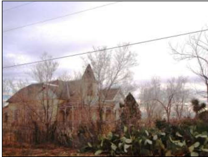
Figure 4.12. Derelict property with overgrown grounds.
