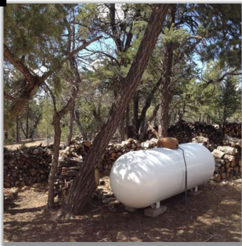
Image 5. Wood piles near propane tanks and other structures increases fire risk
