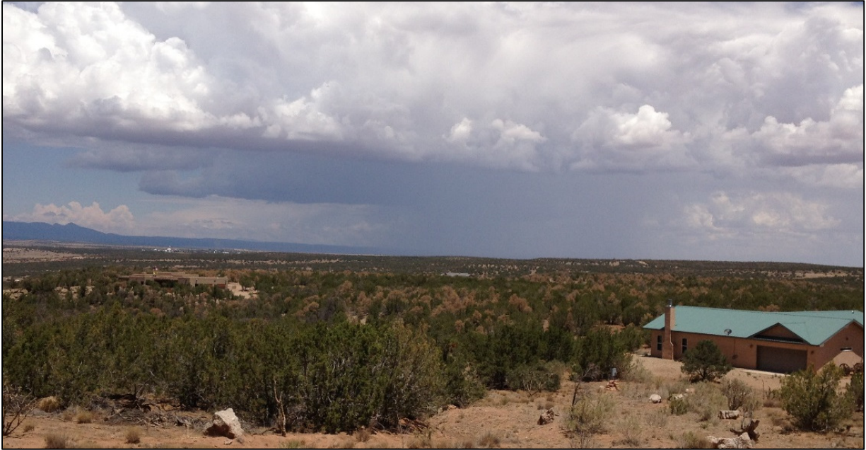
Figure 4.5. Lots of dead fuels within Deer Canyon Preserve, however strict building codes are enforced.
