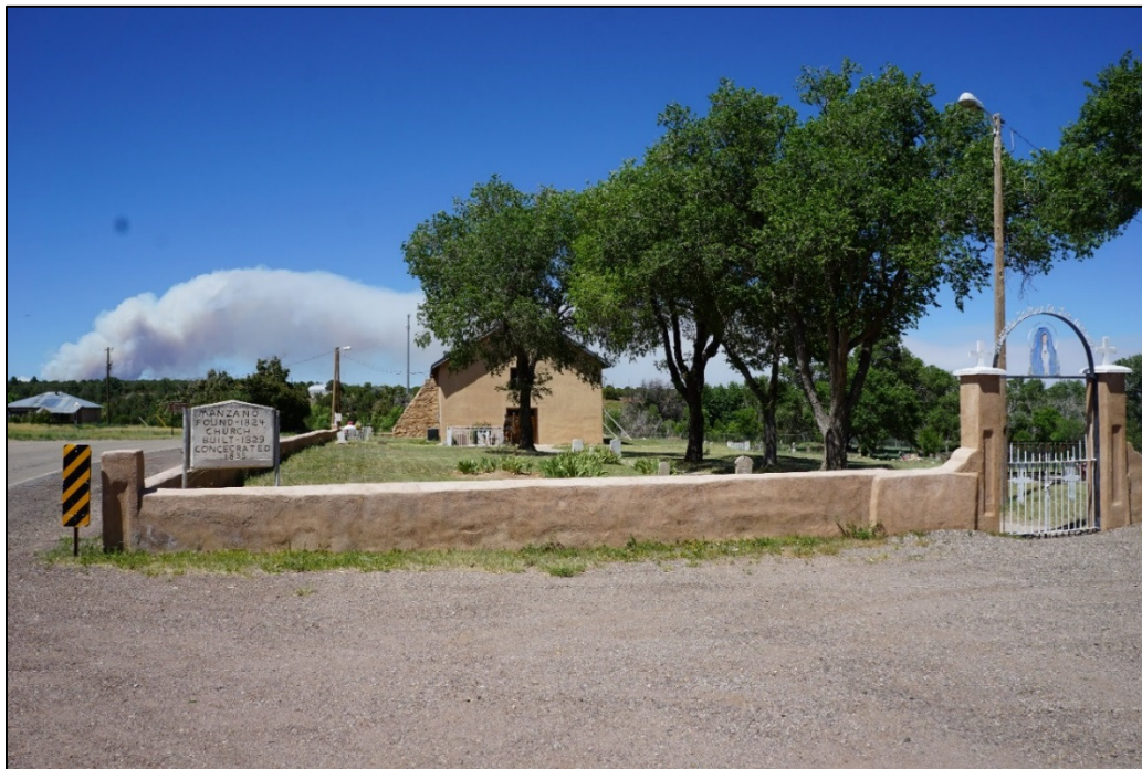
Figure 4.9. Manzano Church with the Dog Head Fire burning in the background. Source: Cody Stropki
