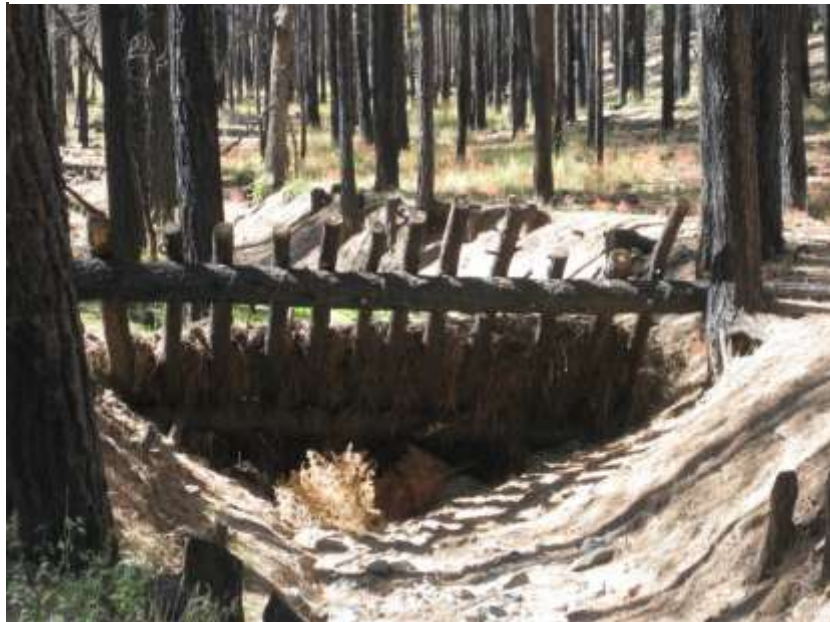
Figure 10. Trash rack constructed with ponderosa pine
