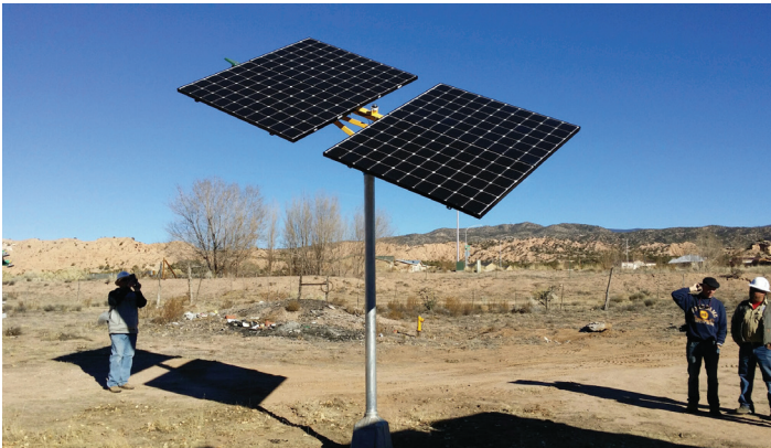
November 2018, Nambe Pueblo – First Installation of PV on a Pole™
