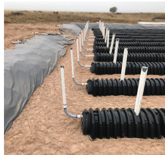
Evapotranspiration bed at Bluewater Lake.
