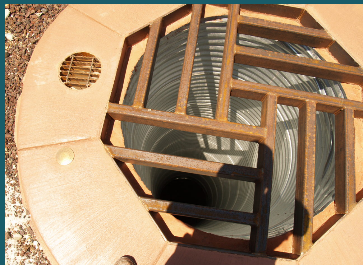
Lloyd Moiola and James Smith Demonstrate the High Tensile Strength Steel Mesh Design Used by NMAML, to Safeguard Several Vertical Shafts at the Lake Valley-II Project
