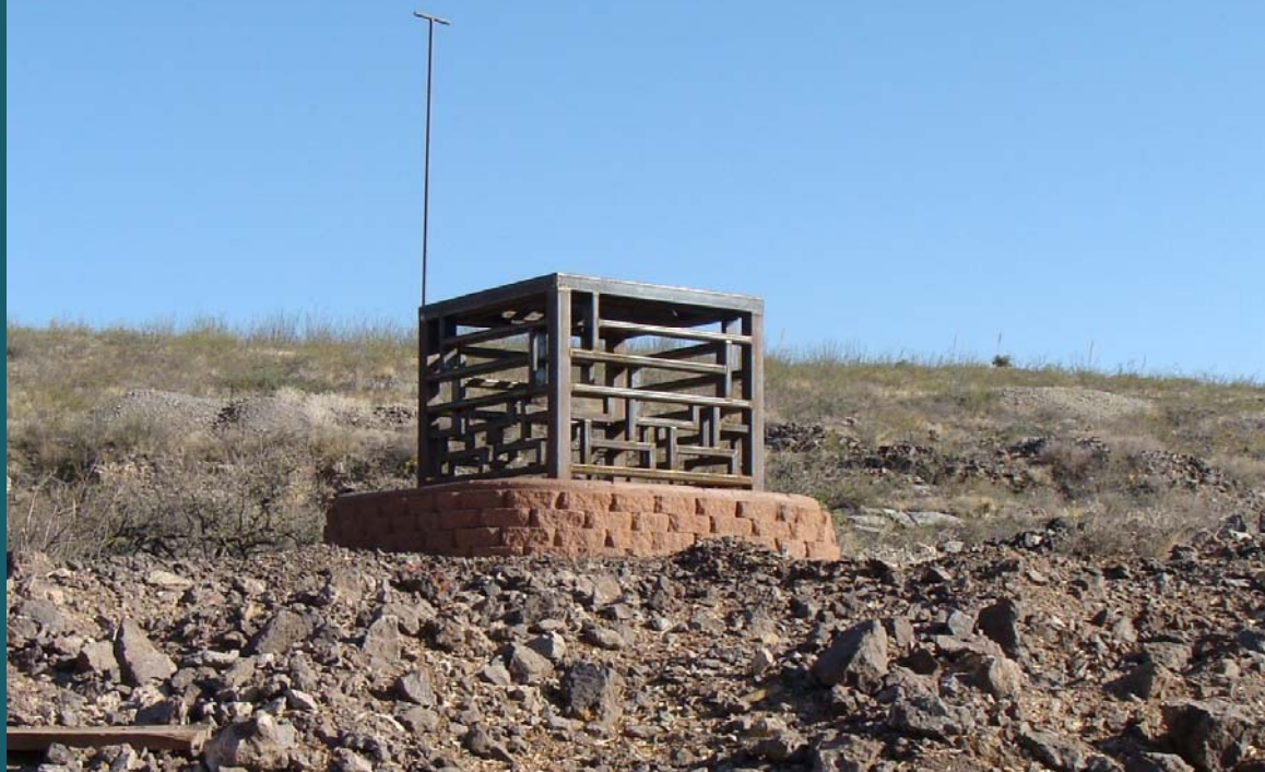
Bat Cupola with Owl Perch - Placed Over Vertical Shaft at Lake Valley-II One of several bat cupola designs by John Kretzmann, NMAML
