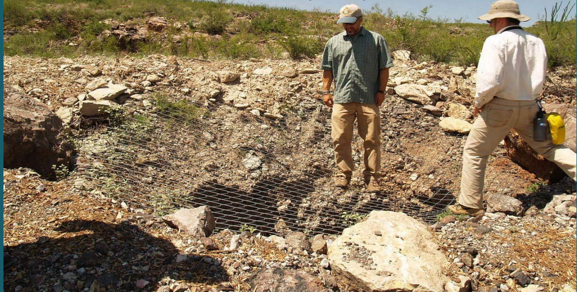
Lloyd Moiola and James Smith Demonstrate the High Tensile Strength Steel Mesh Design Used by NMAML, to Safeguard Several Vertical Shafts at the Lake Valley-II Project
