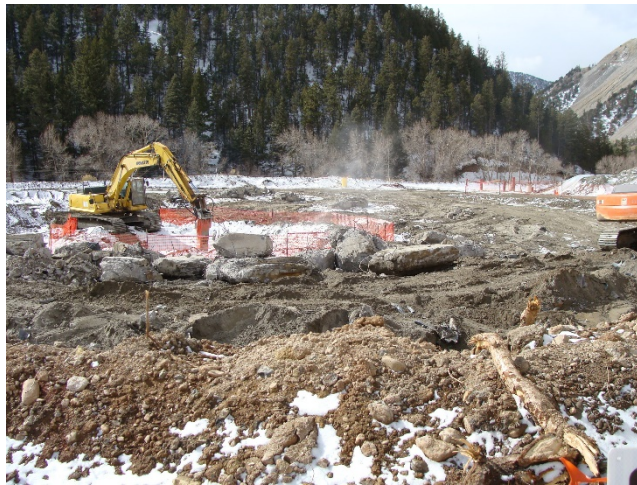
Excavation at the Questa mill during demolition.
