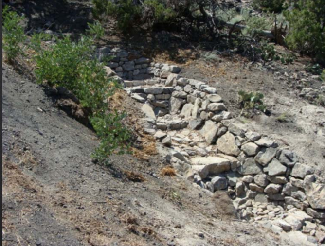
Hand-built step-pool rock channel at edge of larger gob pile July 2014
