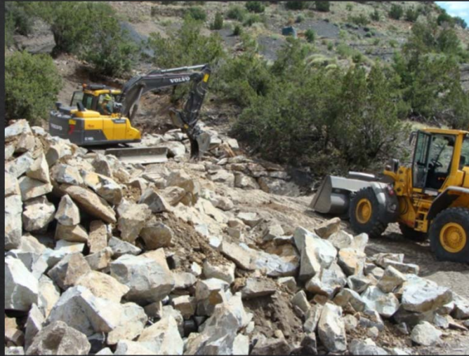
Constructing a machine-built, step-pool rock bypass channel around blown-out gob pile July 2014
