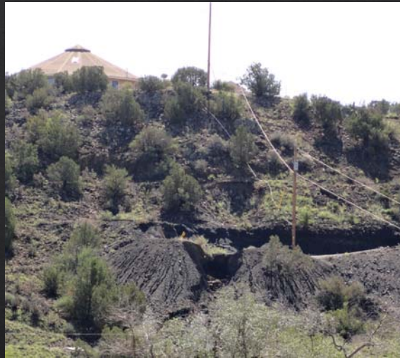
Deeply eroded gob pile above Museum and Icehouse Road. Precast barriers were placed along the driveway above the gob pile to divert runoff to the upper drop inlet
