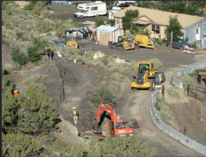
Working in tight quarters to construct a rock bypass channel July 2014
